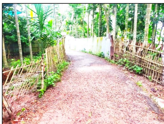
Road-009, Ulipur Pourashava
